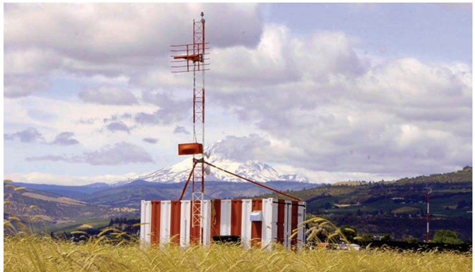
Transponder Landing System
